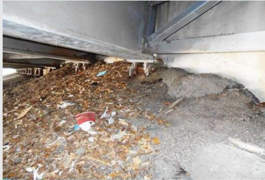
SW ABUTMENT BEARINGS BURIED IN DIRT AND DEBRIS LOOKING SOUTH
