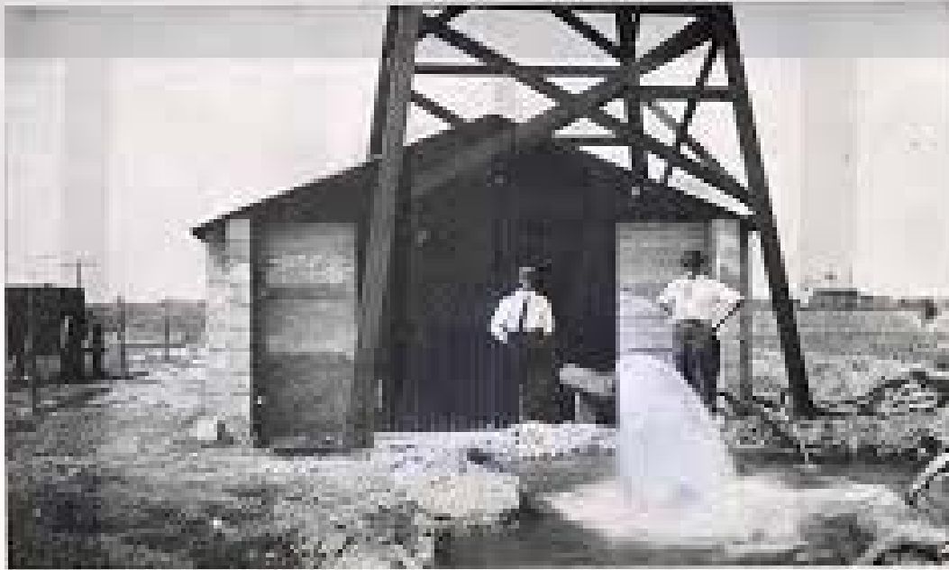
McDonald Irrigation Well, 1000 Gallons per Minute, Hereford, Texas.
